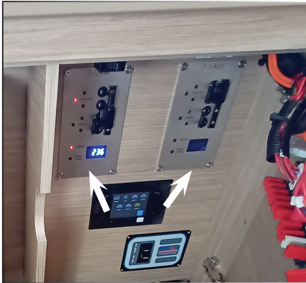
SELECTION PANELS FOR 110 V - 220 V POWER SUPPLY
