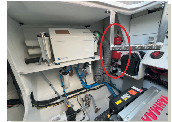
Starboard engine compartment extinguisher
