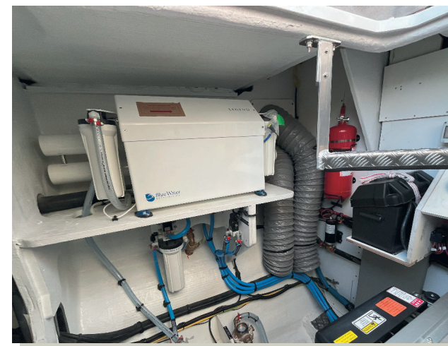
9 STARBOARD ENGINE COMPARTMENT
